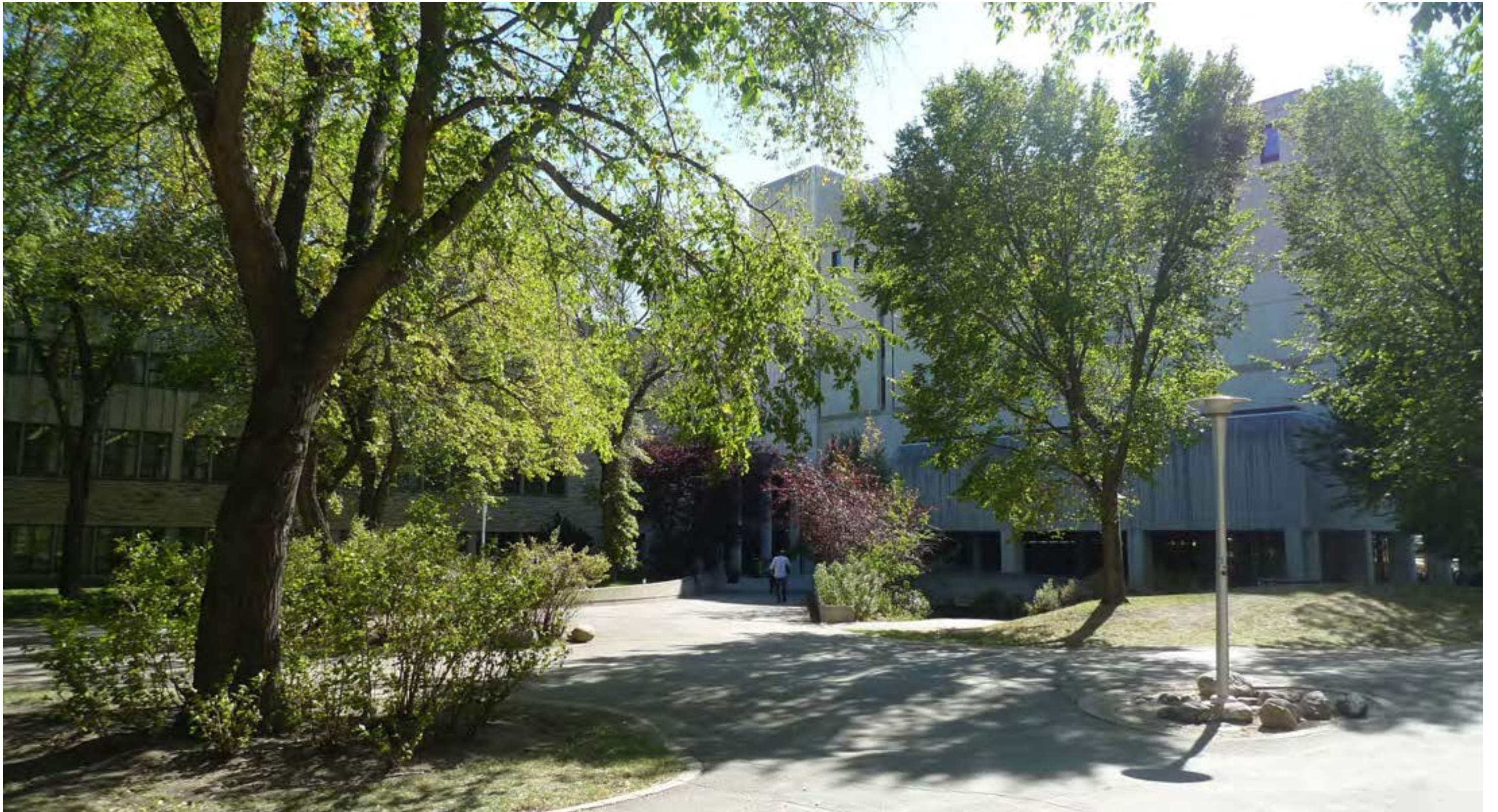
EXISTING LIBRARY NORTH-WEST ENTRANCE
