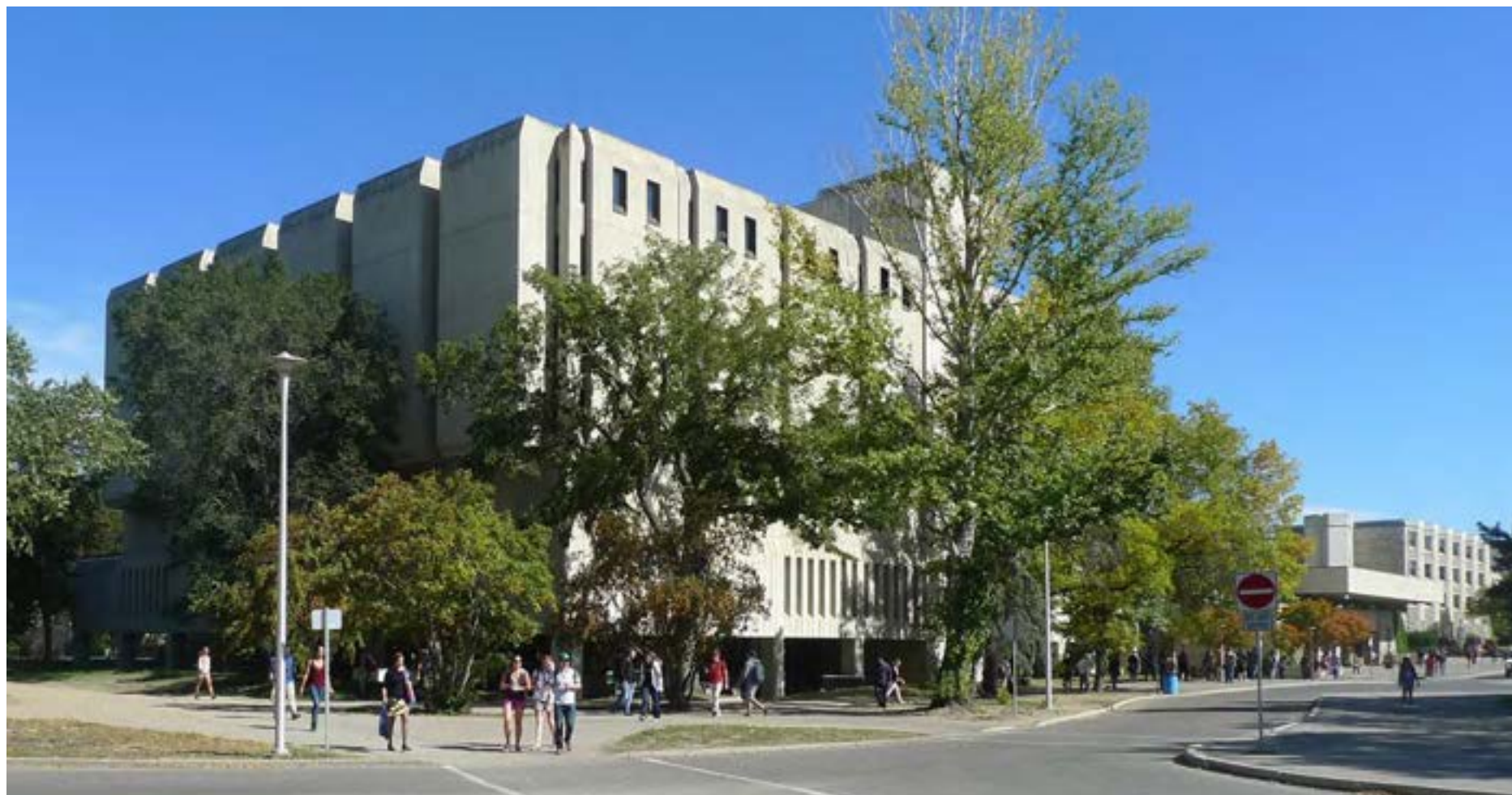
MURRAY SOUTH BUILDING, SOUTH-WEST CORNER
