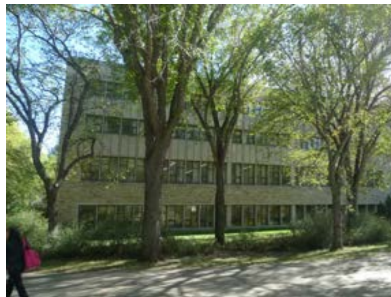
MURRAY NORTH BUILDING
