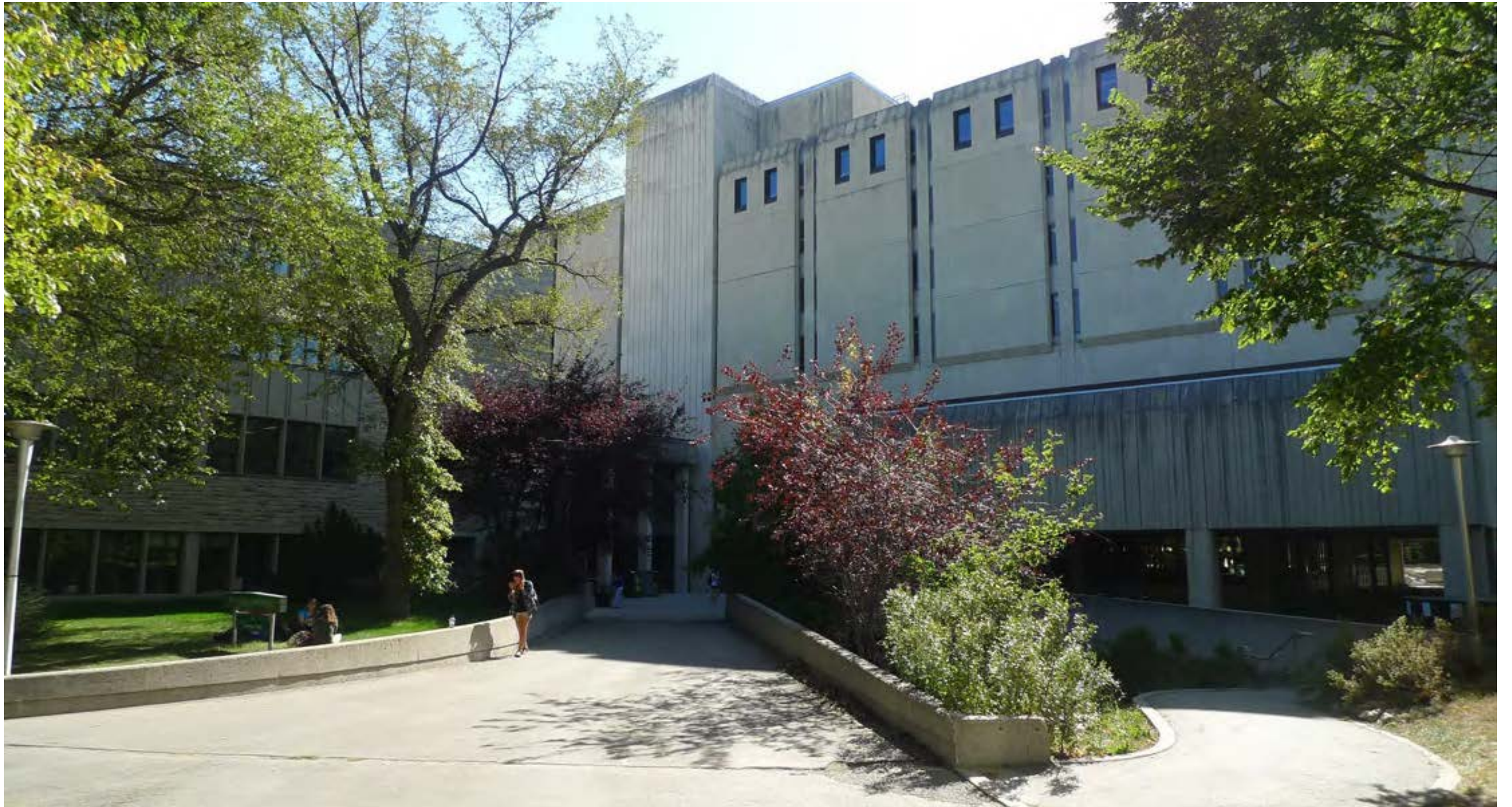
EXISTING LIBRARY NORTH-WEST ENTRANCE
