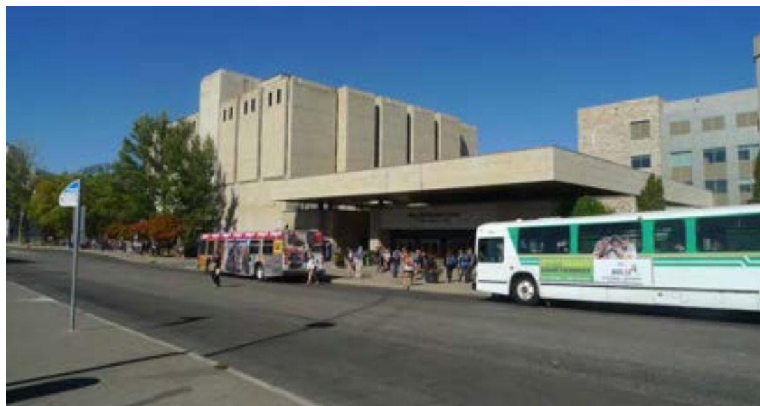
MURRAY SOUTH BUILDING, SOUTH-EAST CORNER
