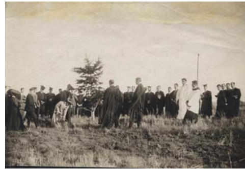
Mrs. Lloyd turned the sod for the present fine stone building. F47 (A-319)
