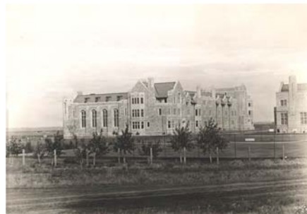
The College of Agriculture, Saskatchewan Hall, girl's residence, and Qu'Appelle Hall (1917), men's residence, before the campus was excavated. 22 F21 (A-736)
