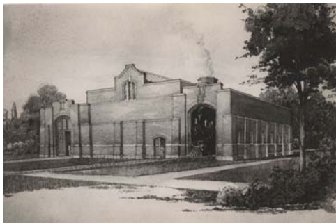
The Power House F18 (A-686)
