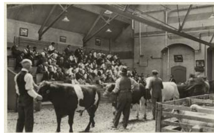
The Interior of the Stock Pavillion, one of the original buildings 21 F20 (A-2239)
